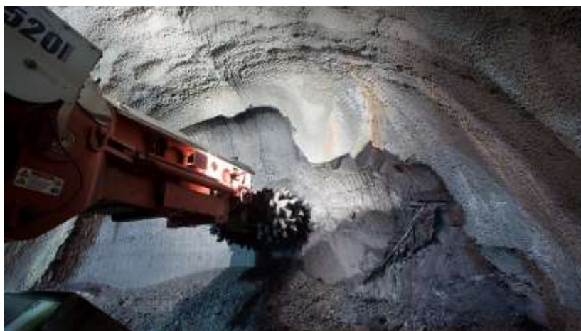
Fig. I-9: Boom Type Machine (B.T.M) in action (image source: Solid Ground Website)
