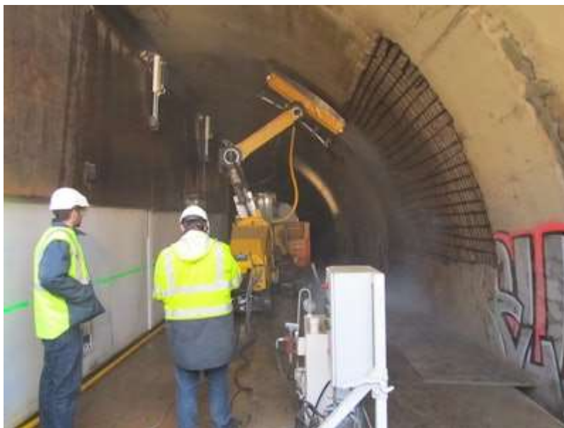
Fig. IV-2: Hydro-demolition process used to selectively remove the damaged and decaying concrete (image source: forconstructionpros Website)
