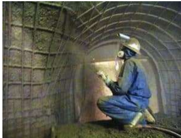
Fig. IV-4: Nozzle man applying Wet Process Shotcrete in tunnel repair (image source: civildigital Website)
