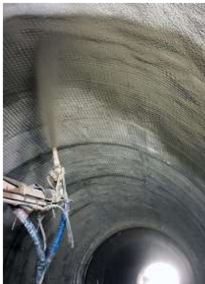
Fig. I-12: Tunnel intrados lining with shotcrete (image source :Strade Autostrade Website)
